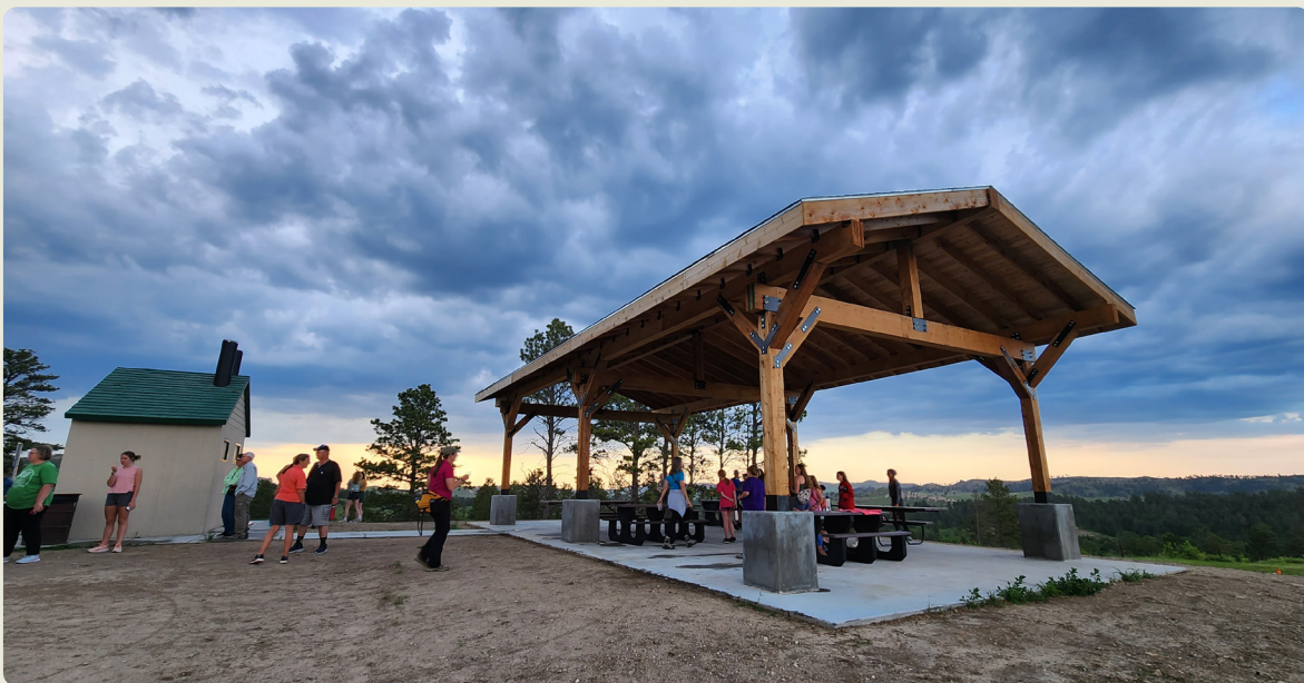
Participants gather at the new Pinecone Shelter for a Wildflower Week event at Chadron State Park. The shelter was made Americans with Disabilities Act-compliant in fiscal year 2022-23 using Capital Maintenance Fund dollars and park cash that included a donation by the Nebraska Game and Parks Foundation.
