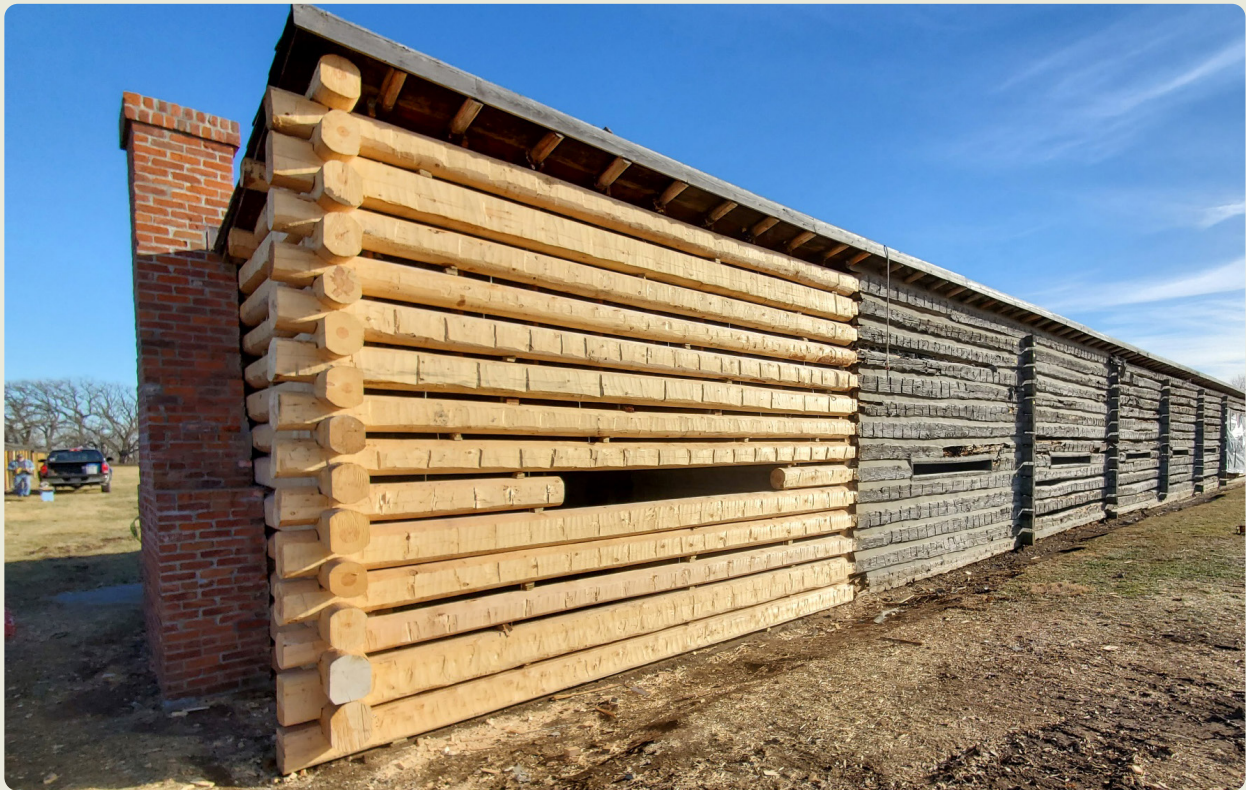
Replacing the logs in Fort Atkinson State Historical Park's historical structures has been a multi-year project funded in part by Capital Maintenance Funds. The park is near Fort Calhoun in Washington County.
