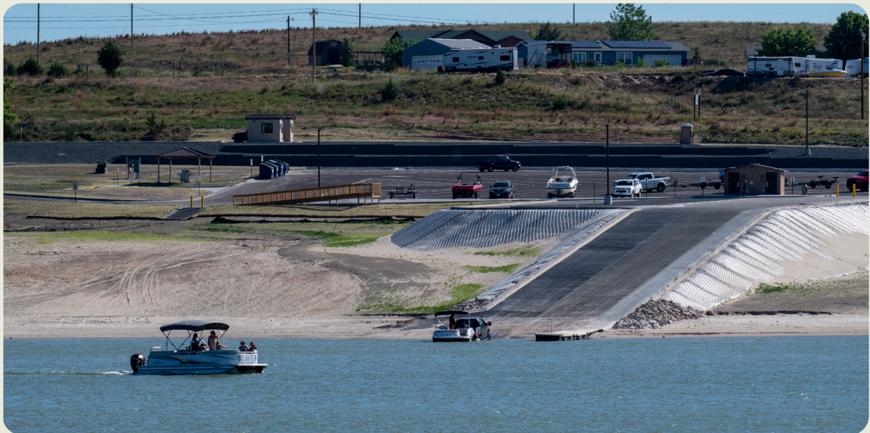
An improved boat ramp, parking lot and Americans with Disabilities Act-compliant ramp in Martin Bay are part of a Motorized Water Trails project at Lake McConaughy State Recreation Area in Keith County. This phase of the project, completed in May 2022, was funded partially by the Capital Maintenance Fund.
