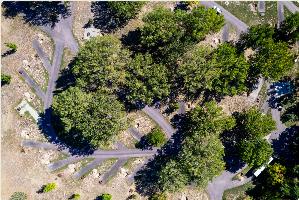
Soldier Creek Campground sites were upgraded to 50-amp service at Fort Robinson State Park in Dawes and Sioux counties. The electrical upgrade was completed in fiscal year 2022-23.
