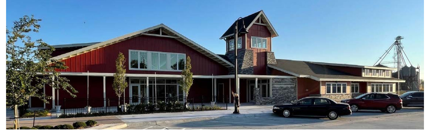
The City of Laurel constructed a new civic center with assistance from a CCCFF grant received through the 2020 Application Cycle.
