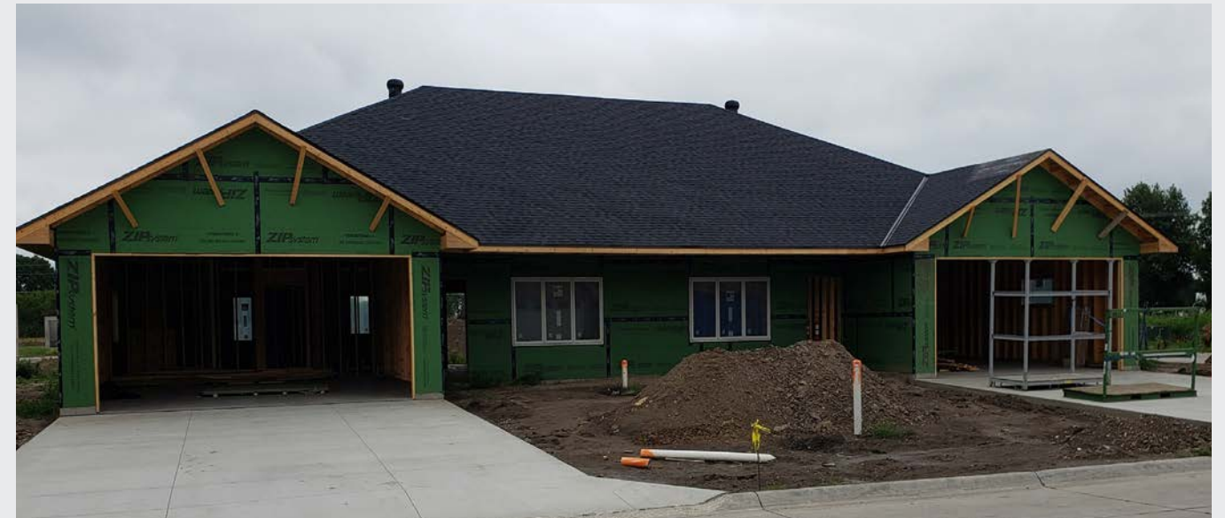
A duplex under construction in the Centennial Housing Project in Columbus.
