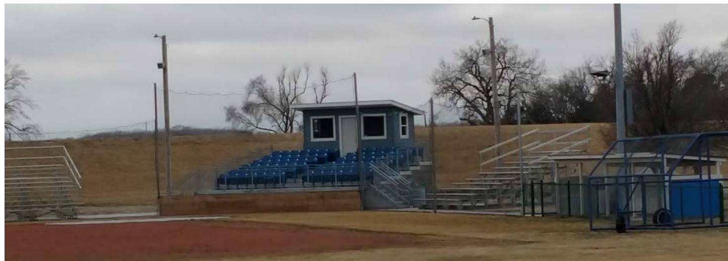
A CCCFF award in Program Year 2020 helped the City of Hooper renovate its baseball field.
