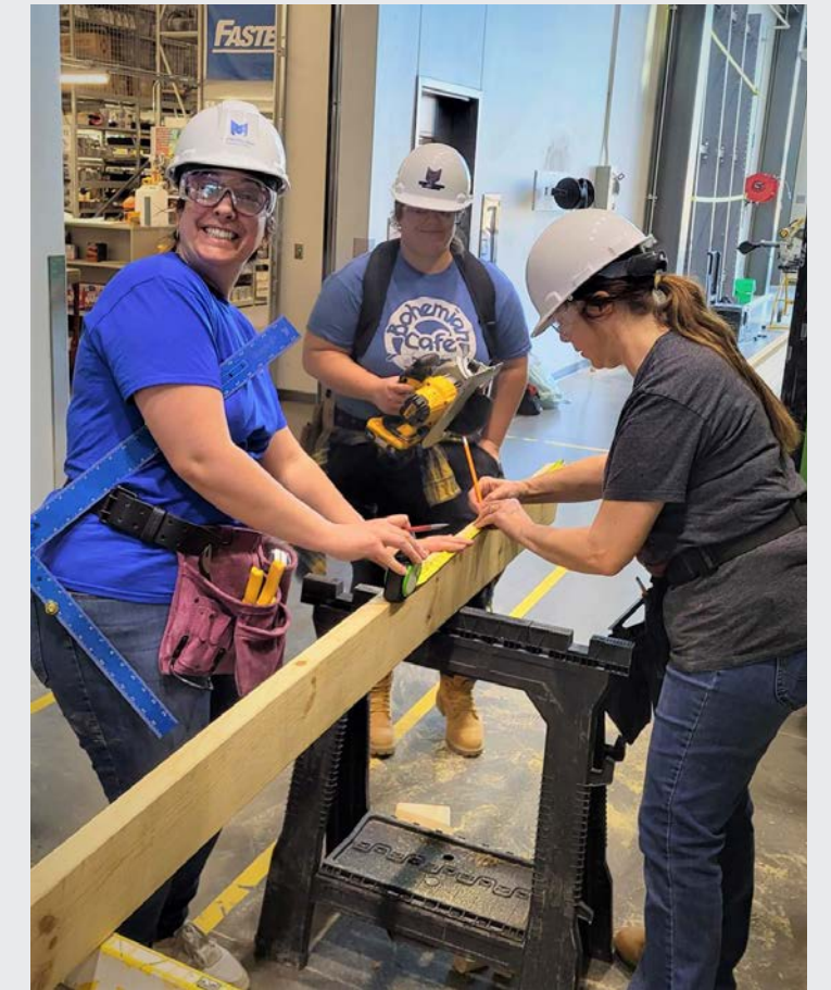
Students take measurements as they construct a home at Metropolitan Community College in Omaha.
