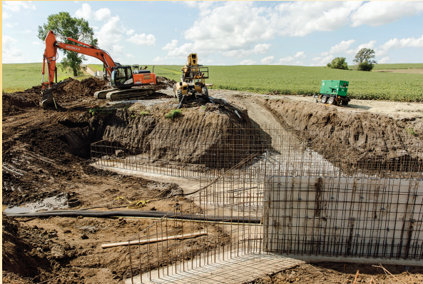
County Bridge Construction Site West of Palmyra
