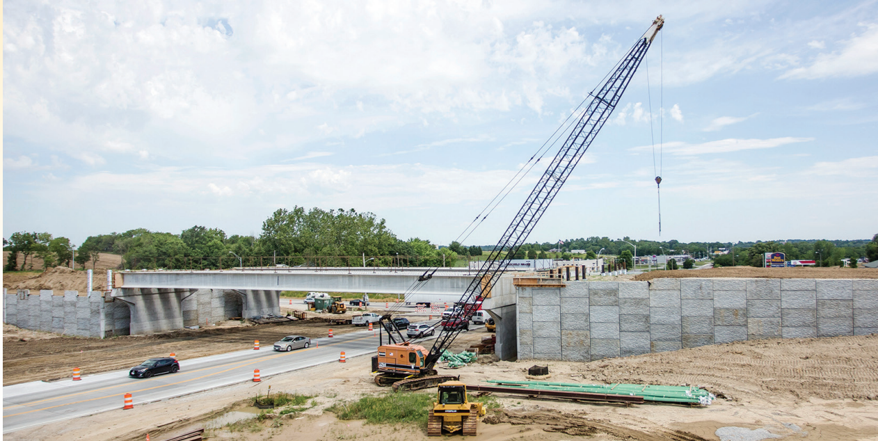
Construction on Nebraska City Project
