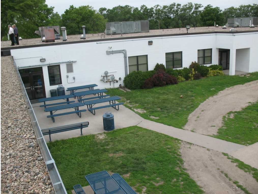
Exterior Courtyard Looking Northwest
