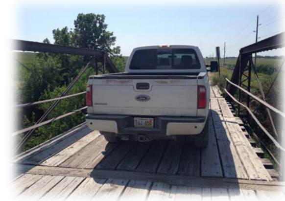
SOME NEBRASKA BRIDGES ARE WIDE ENOUGH FOR A PICKUP, BUT NOT FOR MODERN FARM MACHINERY.
