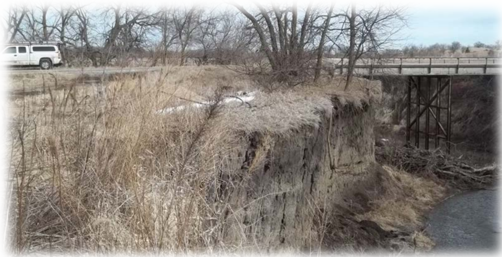
A JOHNSON COUNTY BRIDGE SPANS A CHANNEL WITH STEEP VERTICAL BANKS.
