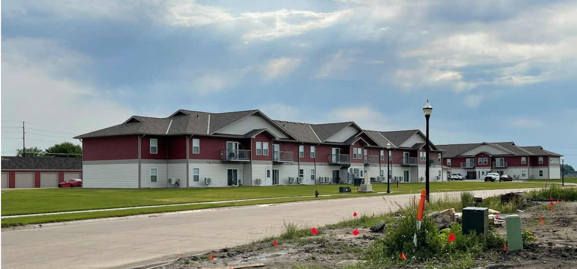
Fountain Springs 55+ apartments
