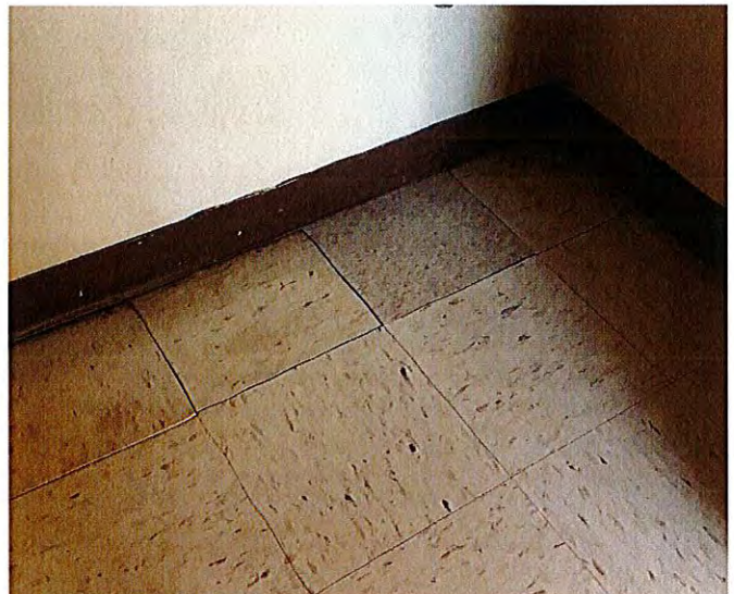
Floors and baseboards
