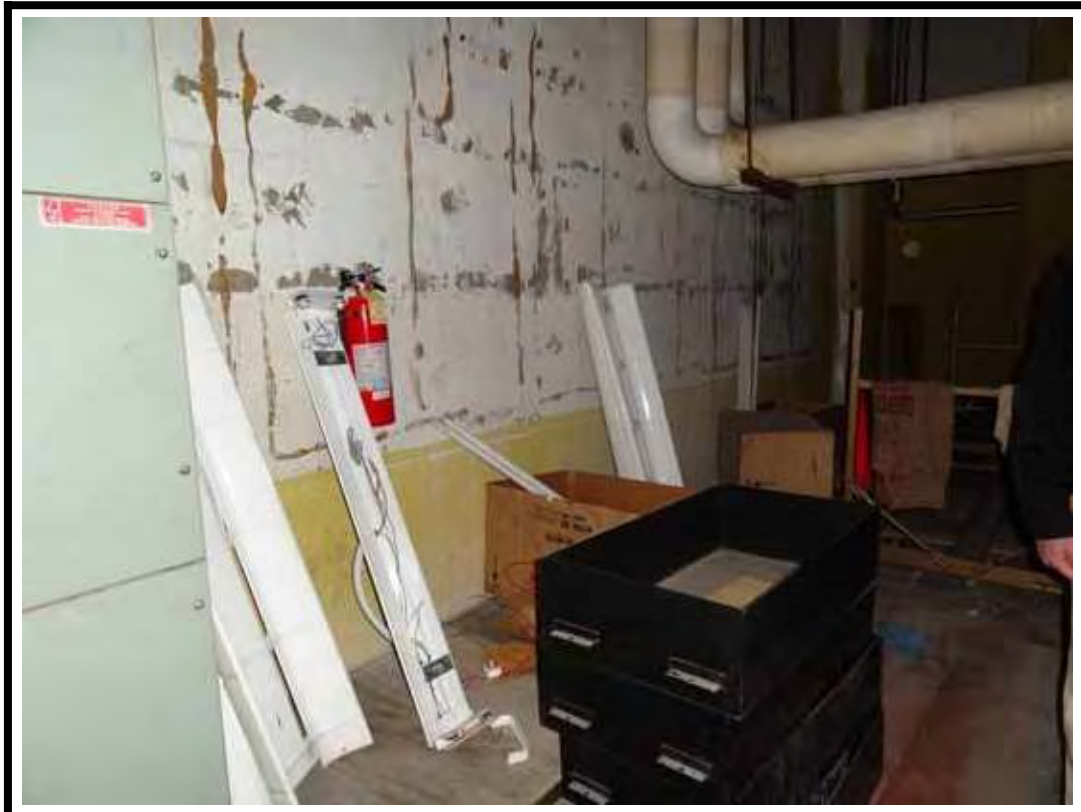
PHOTO NUMBER 49 View of storage in the subbasement.
