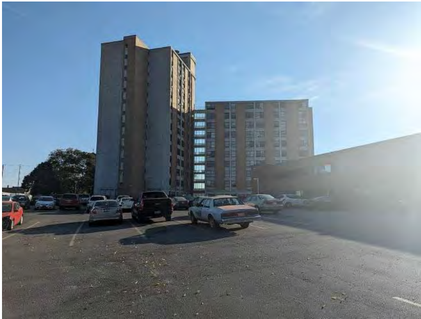
TOWER AND OFFICE - NORTH
