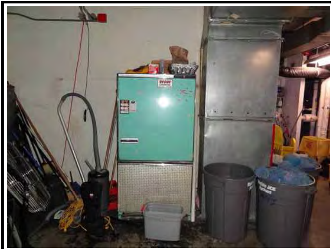
PHOTO NUMBER 11 View of janitor's closet in the Arena.
