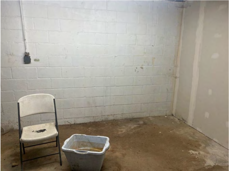
Existing basement area that will be excavated to provide a new entrance to the Community Center
