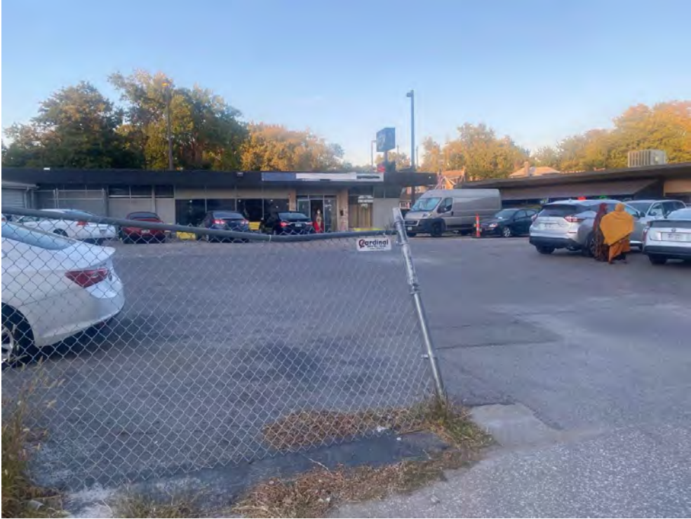
Existing parking area that would be demolished and used to create outdoor space for the Community and Cultural Center
