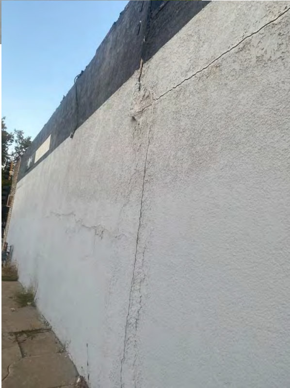
Current conditions of exterior of the building
