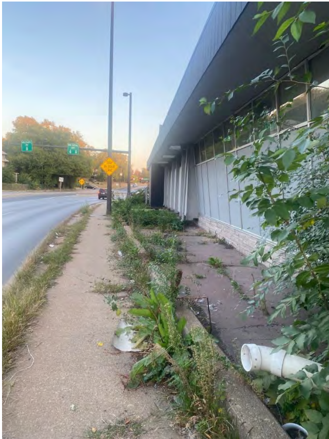
Current conditions of exterior of the building
