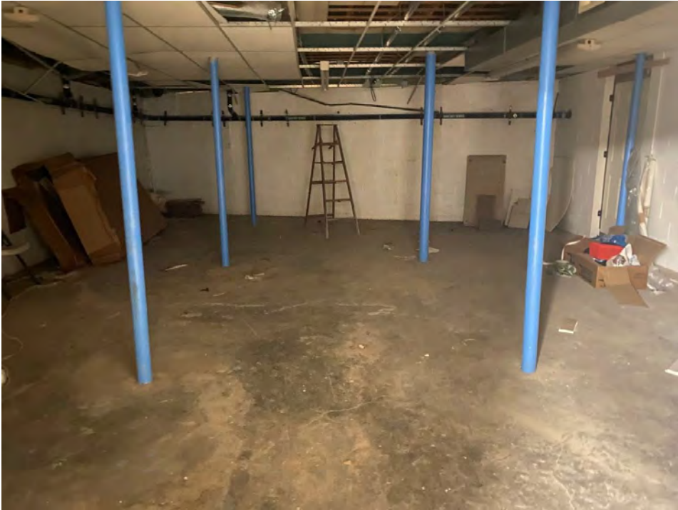
Existing basement area that will provide space for the women's gym.
